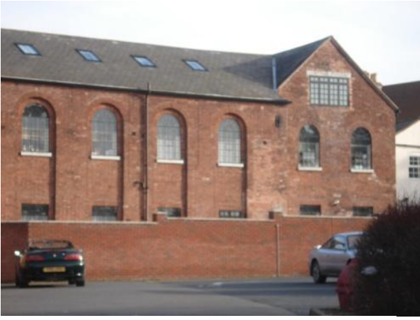
Fig. 5: , Former chapel and factory, Wellington
