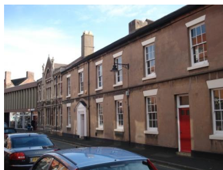
Fig. 10: Existing library, Wellington
