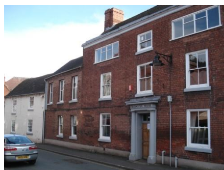
Fig. 11: Edgbaston House, Wellington – all three sections of which are earmarked for demolition under the current plans
